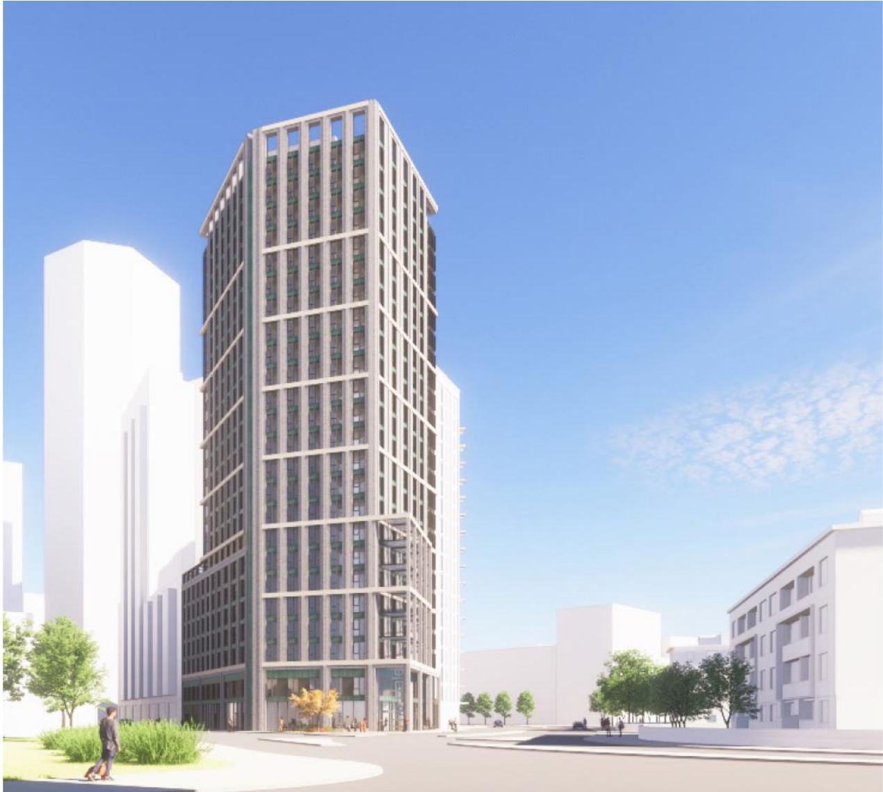
View from Down Lanes Park looking south
